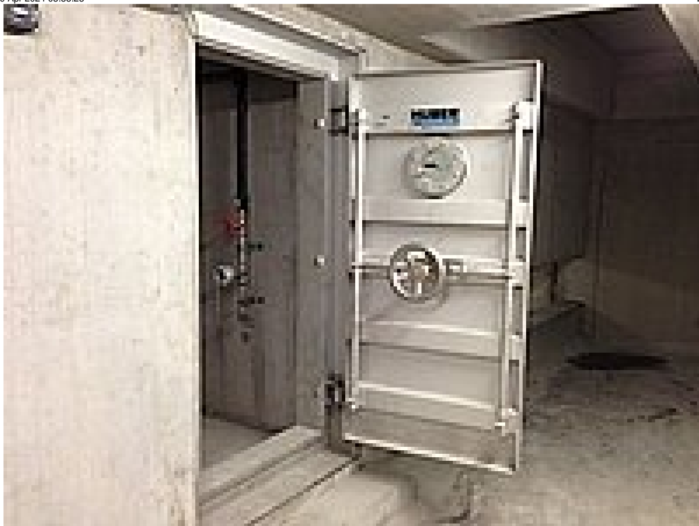
Pressure door with central lock
