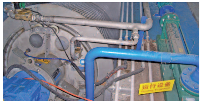
Screenings removal by pump (e.g. eccentric screw pump)
