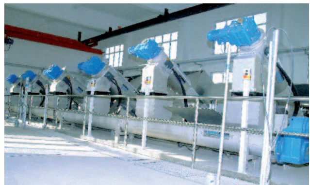
Fine screening with a ROTAMAT® Membrane Screen RoMem ideal for installation in a channel
