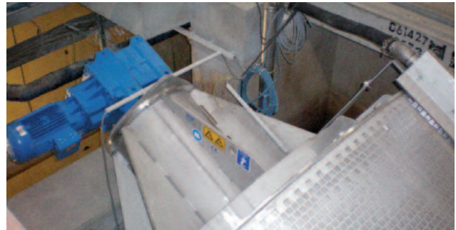
River and sea outfall application: ROTAMAT® Membrane Screen RoMem liquid for wastewater screening
