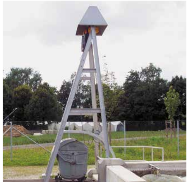
On the HUBER Basket Screen CageLift, the electric lifting mechanism is mounted above the channel or pump shaft, so that the screenings can be discharged directly into a container.
