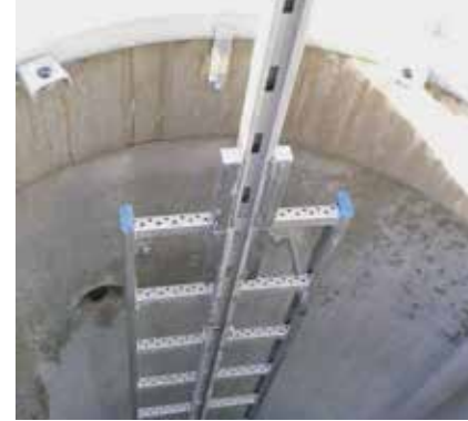
HUBER safety access ladder with fall protection.
