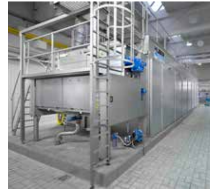
HUBER Belt Dryer BT for sewage sludge drying up to > 90% DR.
