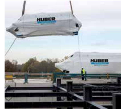
A HUBER Disc Dryer RotaDry® during installation on site.
