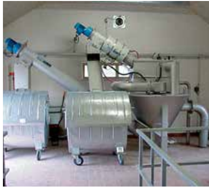
Complete headworks in a single, enclosed and compact unit ideal for small plants.
