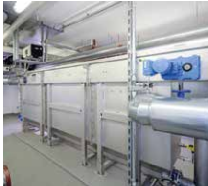
RoWin Heat Exchanger for energy recovery.
