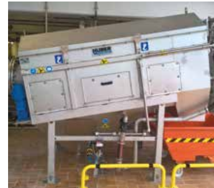
Washing of contaminated grit with the versatile HUBER Wash Drum RoSF9.
