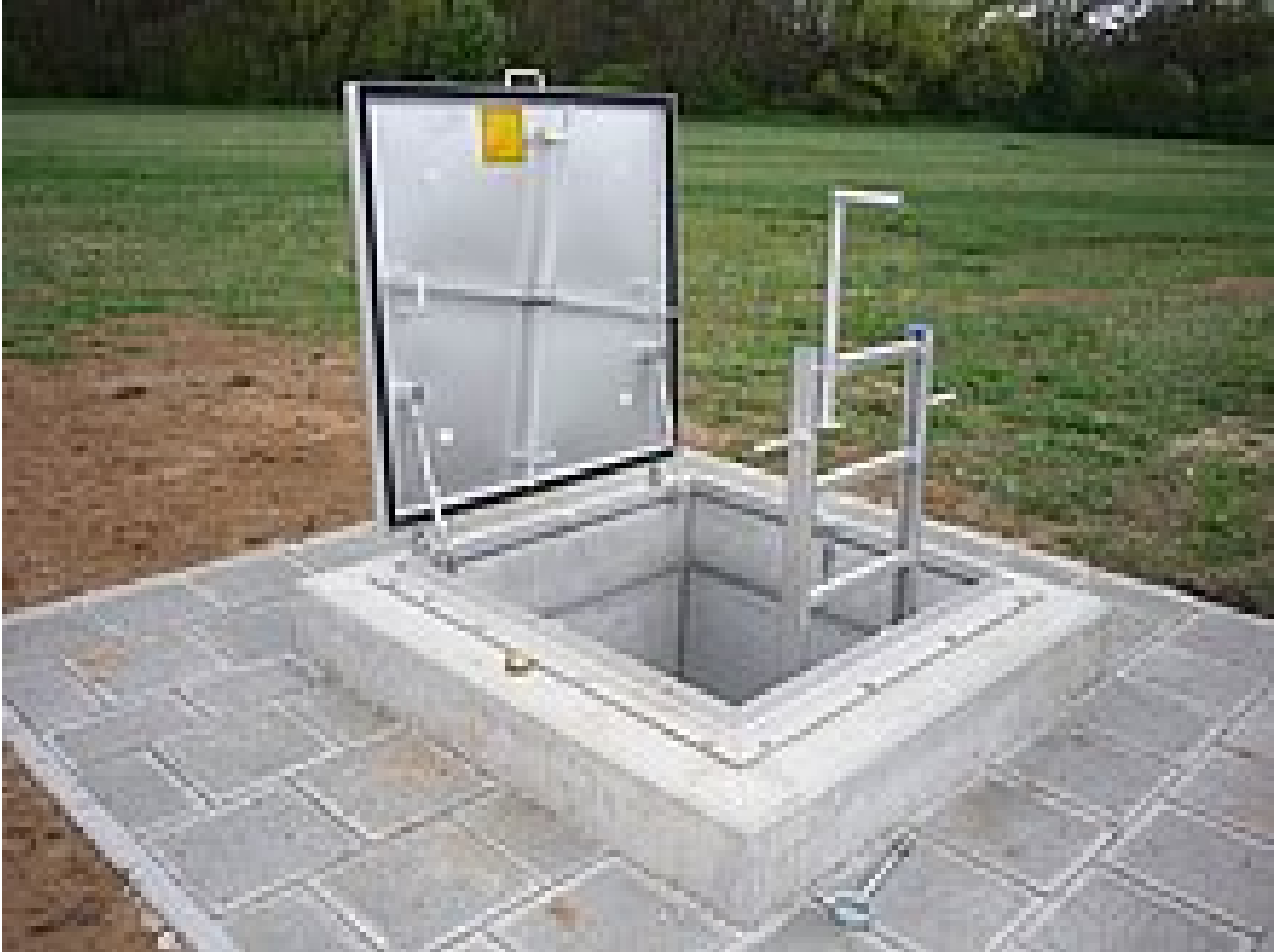
Newly refurbished manhole
