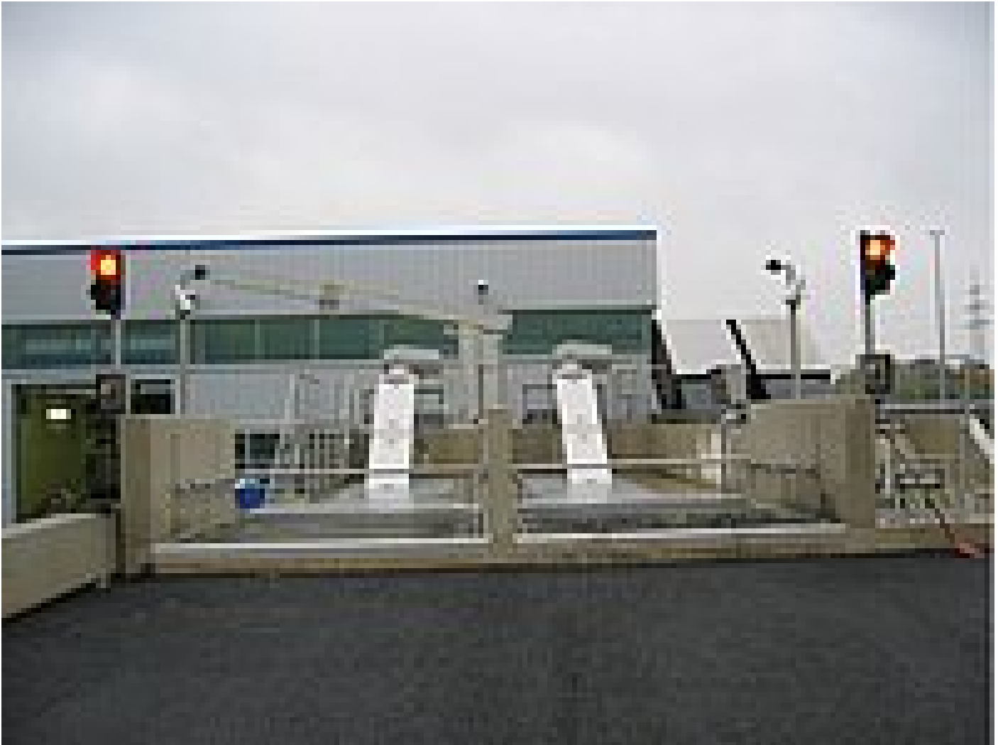
Pair of 20 m 3 slurry receiving tanks with Ro 8 screw conveyors
