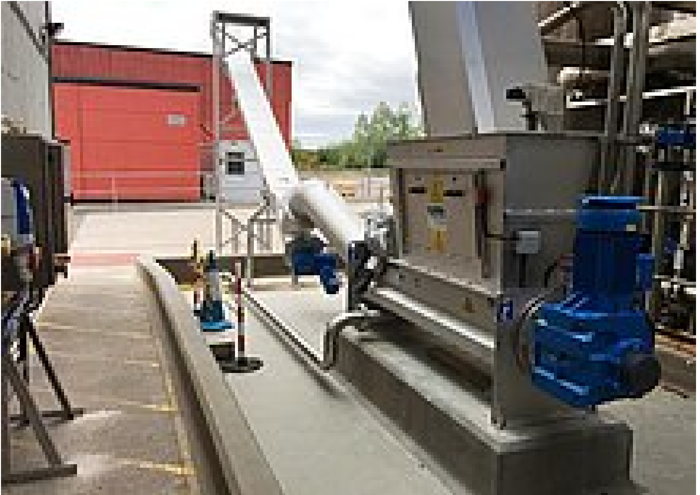
HUBER Screenings Wash Press WAP® L 6 compactor and HUBER Screw Conveyor Ro8 T conveyor
